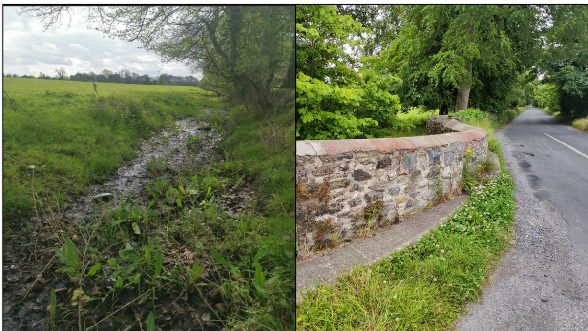
Figure 4-4: Drainage Ditch (Left) and Stone Walls and Other Stone Work (Right).
